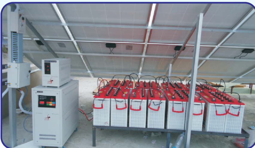
Installation of 8KW Solar Off grid system at Rajasthan.
